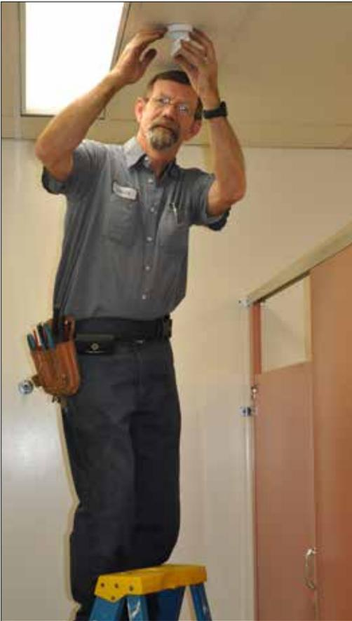
Chuck Dazey installs a light sensor in a bathroom at the Whipple-Dale Centre. Potential energy savings from sensors could be 40 percent. Sensors will be installed in all building common areas by spring of 2013.
